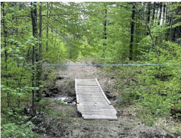
Example of bridge crossing with disconnection practice
