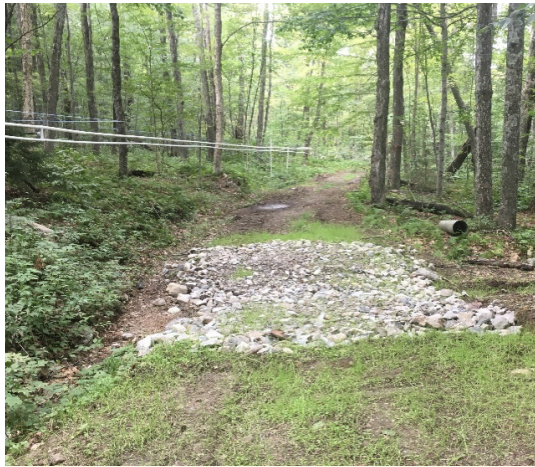
Wet section of trail hardened with stone.
